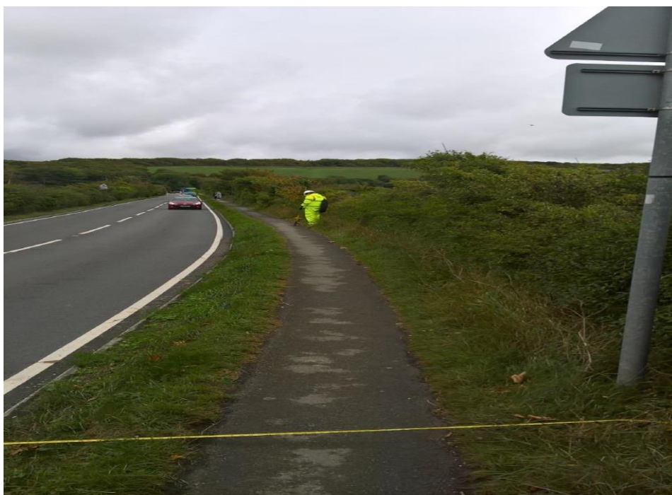
Figure 5. Existing footway from West to East
