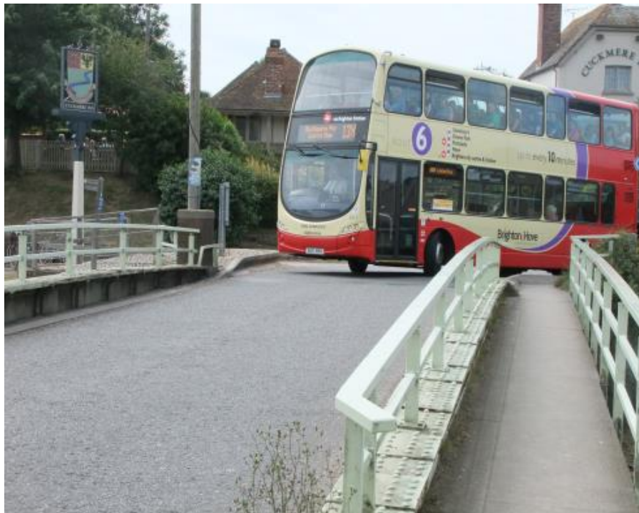
Figure 3 Photo of bus squeezing around the bend from West side of 1 way bridge.
