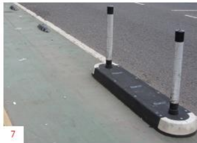
7. 130mm diameter wands on a satellite island
