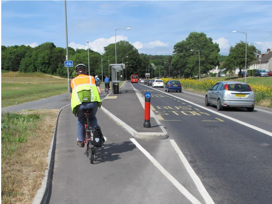
3.1.13 Bus stop boarder with material buffer (Lea Bridge Road)
