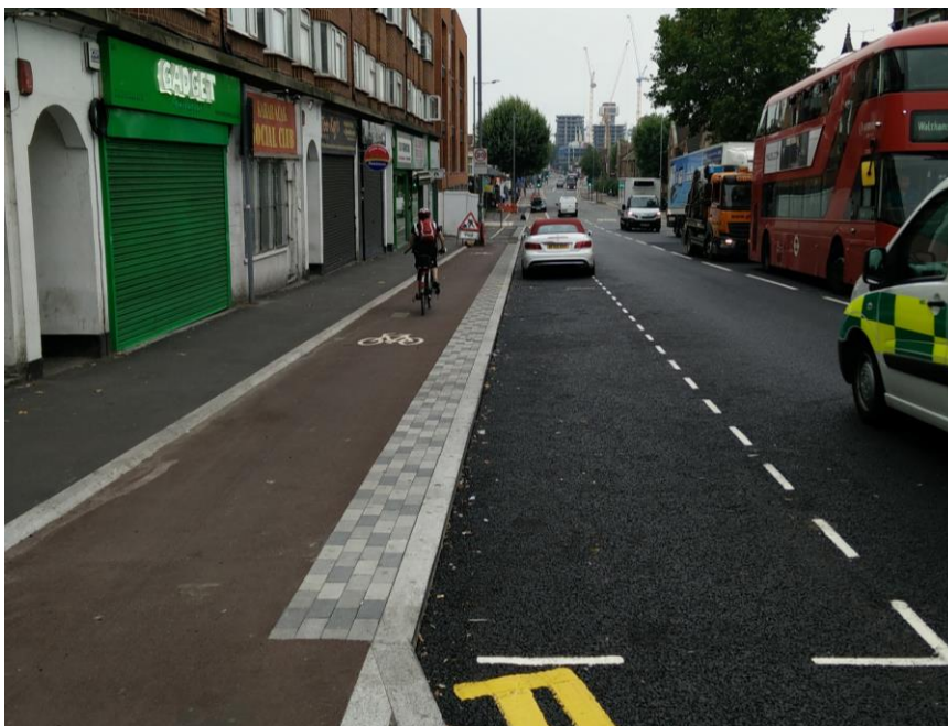
3.1.16 Preformed road hump at garage exit (Blackhorse Lane, Waltham Forest)
