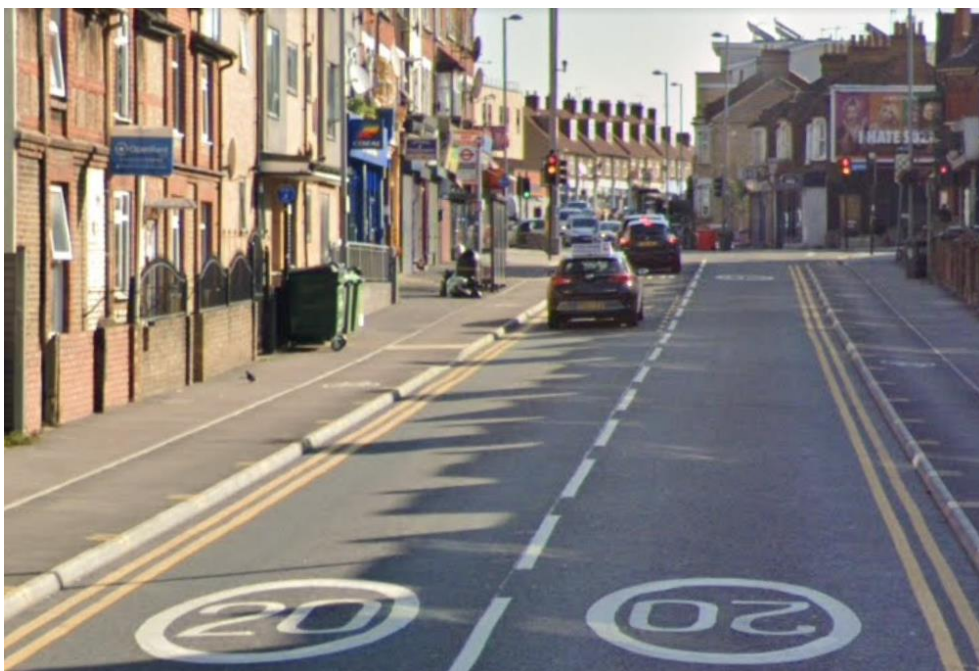
Footway level cycle track with demarcation paving
