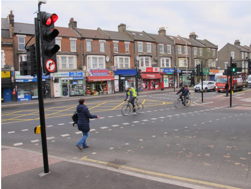
3.1.9 Pedestrian and cyclist crossing at signal junction
