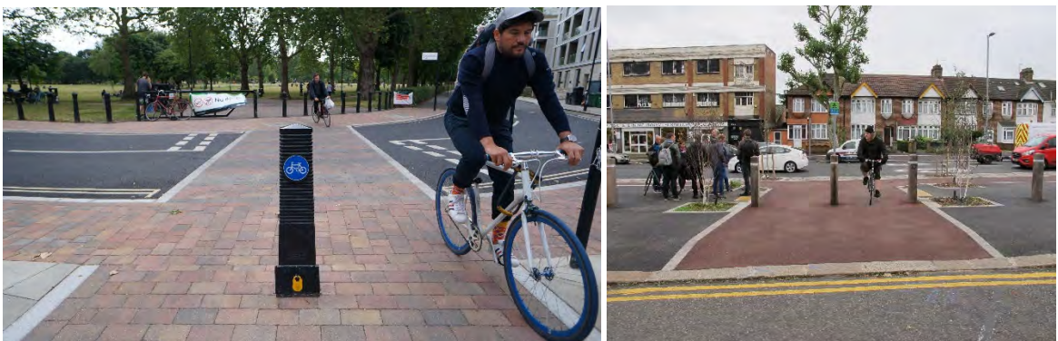
Figure 4-16: Combined informal crossing and modal filter (Downs Road, Hackney), and Modal Filter installed with cycle access (Grove Road, LB Waltham Forest)
