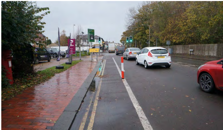
Figure 2-2: EATF Light Segregation on St. John’s Road (A26)
