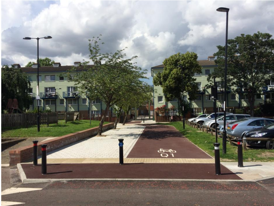
3.1.11 Short section of constrained facilities with de-cluttered footway (Markhouse Road, Waltham Forest)
