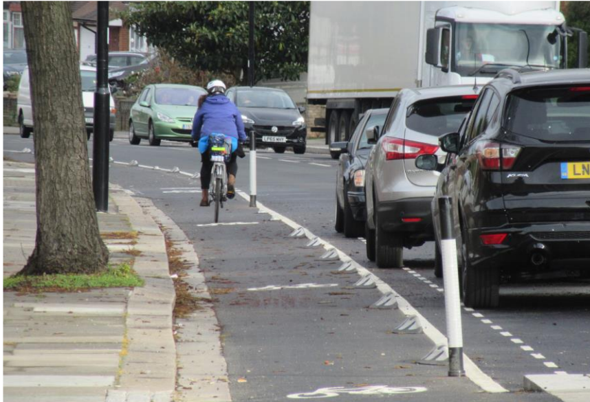
3.1.4 Footway level cycle tracks (Forest Road, Waltham Forest)
