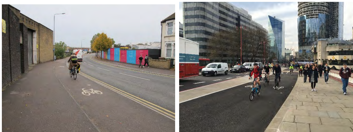
Figure 4-14: Blackhorse Lane (left) has installed narrow cycle tracks alongside the existing footway with a small kerb upstand, and Blackfriars Bridge (right) has installed bi-directional cycle tracks
