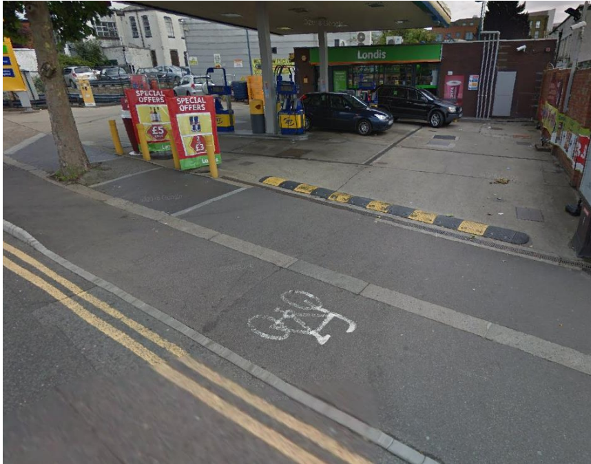
3.1.17 Offset zig-zags with light segregation (Forest Road, E17)
