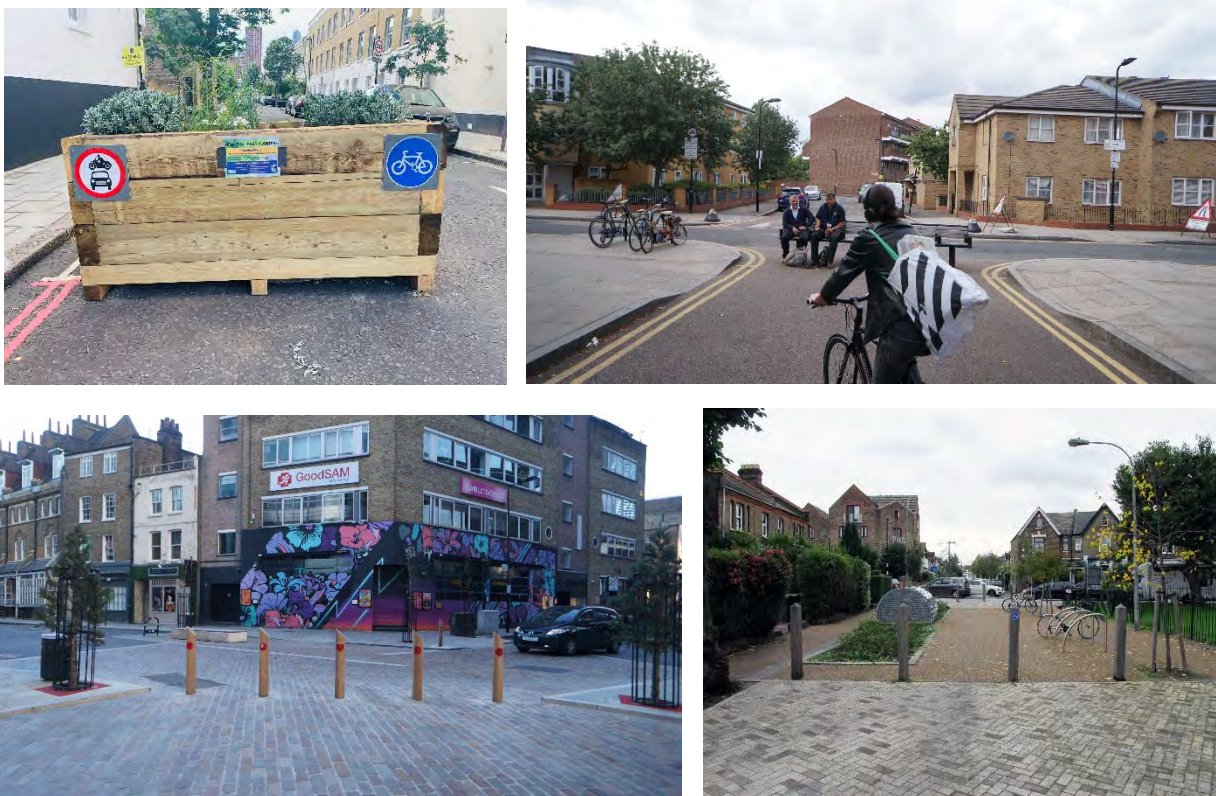
Figure 3-2: Photos from existing LTN schemes and the modal filters used to enforce the closures
