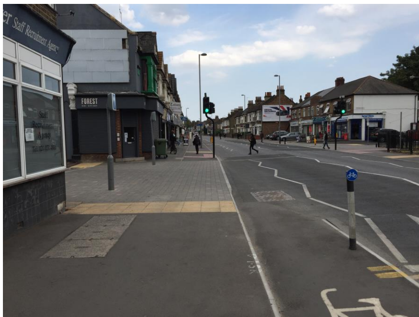
3.1.18 Blockwork used at continuous footway
