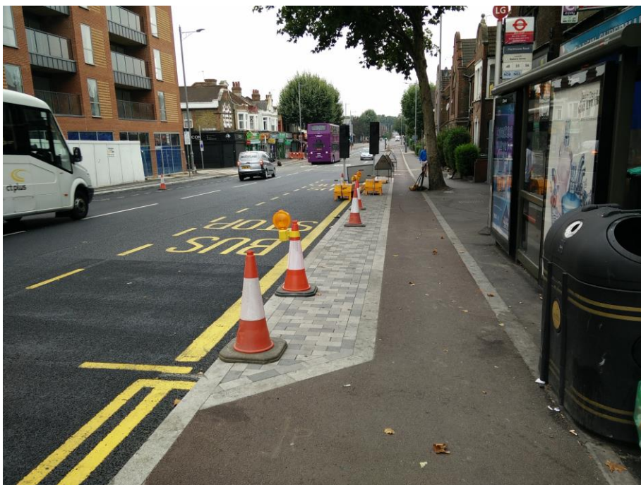
3.1.14 Bus stop boarder (preferred 1:20 ramp for transition) (Enfield)
