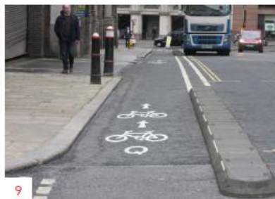
9. A 'defender' unit (as used on West Smithfield)
